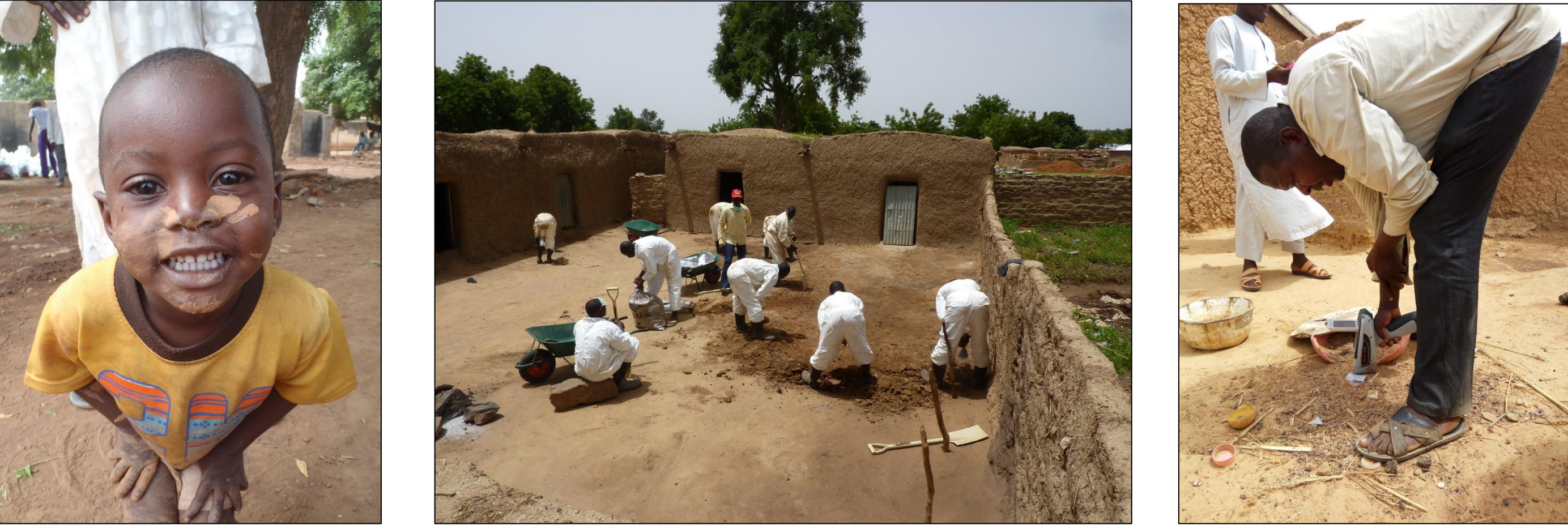
Figure 1. (Left to right) Incidental ingestion of soil and dust is a significant source of children's exposure to environmental contaminants; remediation crew removing contaminated soil in a compound; Zamfara Environmental Sanitation Agency using XRF to measure lead in compound soil.
